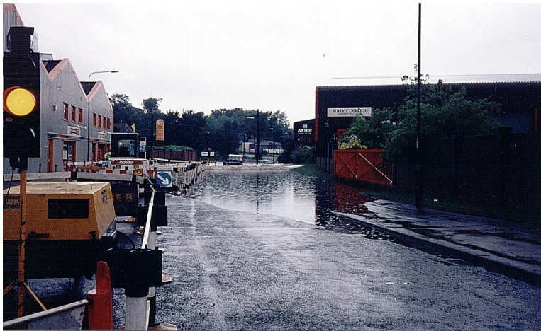
Holywells Road – floods several times per year.
