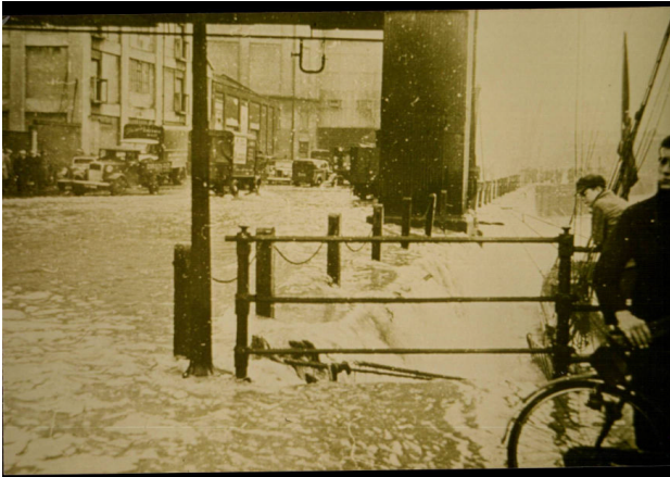
1939 Floodwater from river Gipping spilling into wet dock at Albion Wharf
