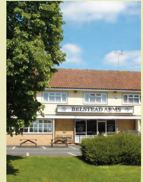
Ellenbrook Green Local Centre
