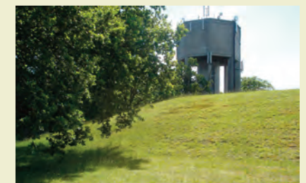
Stone Lodge Lane West water tower and reservoir
