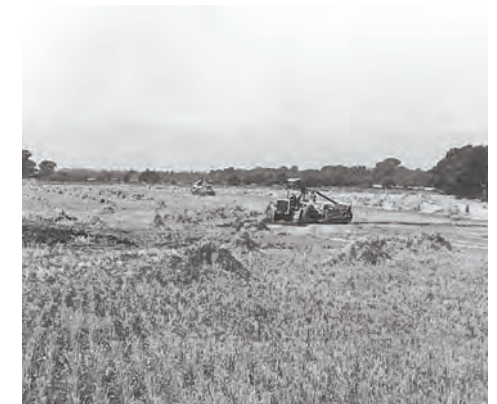
Grading of farmland in preparation for the construction of phase 1 of the Chantry housing estate (early 1950s)
