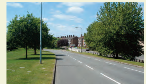
Birkfield Drive. The road is set within a broad landscaped strip originally intended for a dual carriageway - it even has an underpass.
