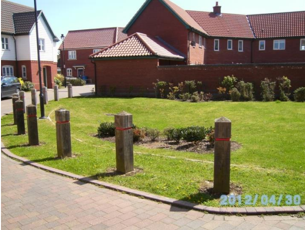
Landscaped shallow infiltration basin with a soakaway below, at low point on road, close to source – sited on inside of bend in visibility splay. Posts keep vehicles out
