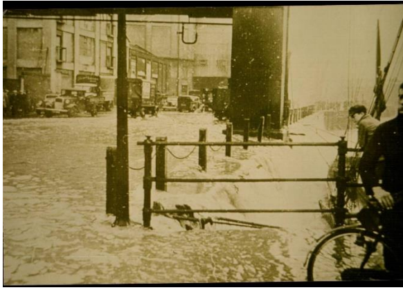
Figure 3-2 1939 Floodwater from river Gipping spilling into wet dock at Albion Wharf
