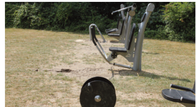
The purchase and installation of four outdoor gym equipment units
