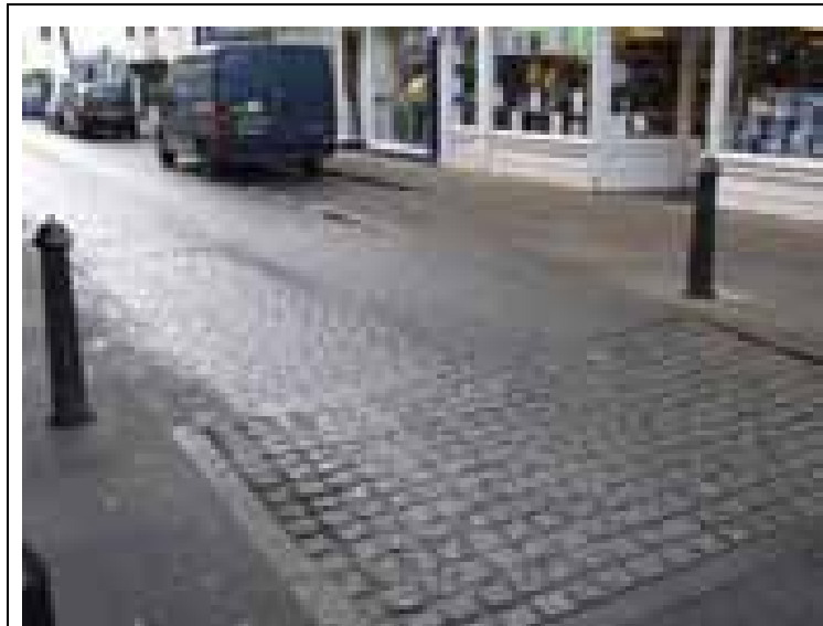
Photograph 2 – Granite setts which disrupt cyclists
