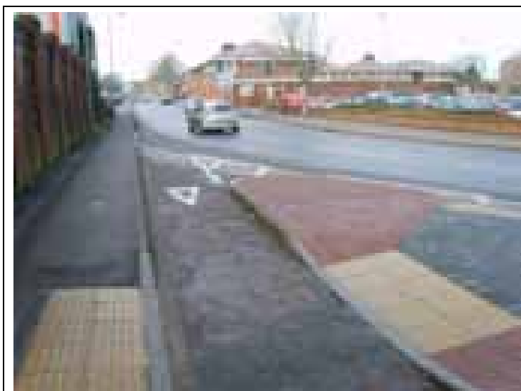
Photograph 5 – Grafton Way, end of existing cycle route at the Commercial Road junction
