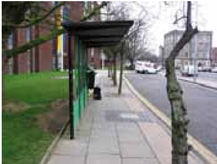
Photo 19: Crown St Coach Lay by
