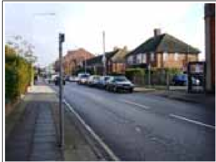
Photograph 4 – The northern footway on Rope Walk
