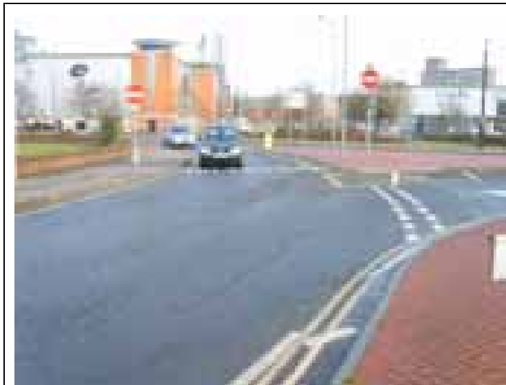
Photograph 6 – Location of proposed northwest toucan crossing on Commercial Road
