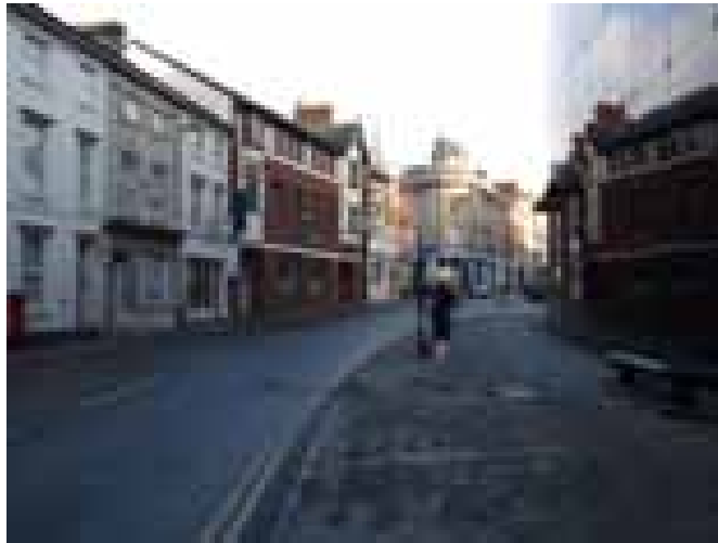
Photograph 6 – Princes Street, looking North, next to Grade 1 Listed Willis Building
