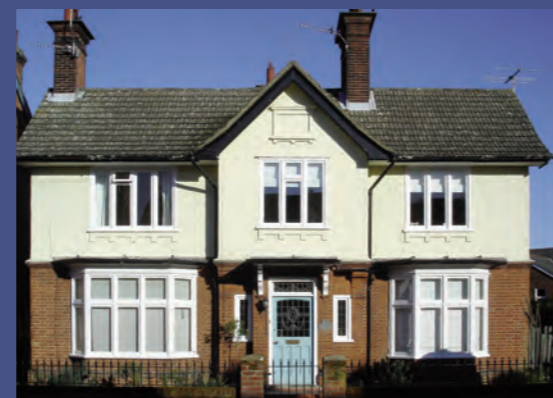
Top: Detached house on Tolworth Road
