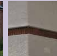
Red brick detail line through white painted render.
