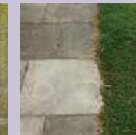
Grass verges: important contribution to the streetscape.
