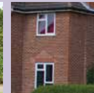
Dominant red brick character with brick work detailing.
