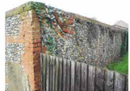
b. Red brick and flint walling
