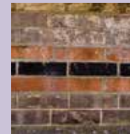
Contrasting red and black brick course detail.
