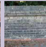
Weathered buff brick with red brick footing detail.
