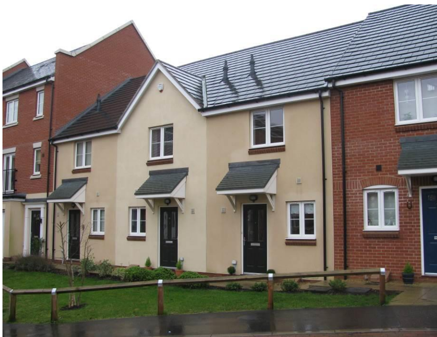
New homes at Meridian Drive, North-East Ipswich
