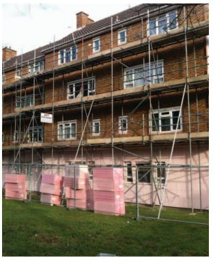
External Wall Insulation is applied to the façade of the building
