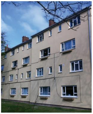
The insulation is rendered over and window boxes are replaced
