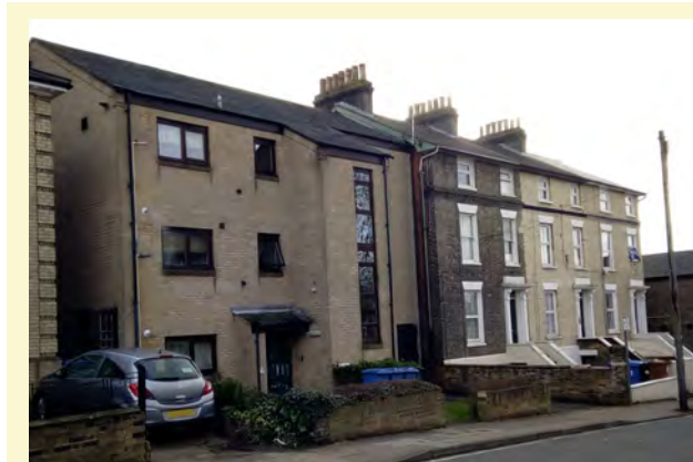
Burlington Road: This image illustrates the introduction of unsympathetic development which does not respond to the character of the area, whilst the terrace shows the impact of brick cleaning from over cleaned masonry which awkwardly contrasts the natural patina of the remaining brickwork.
