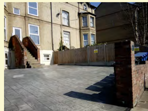
London Road: Loss of well planted front gardens for hardstanding to accommodate car parking erodes the suburban character of the area.
