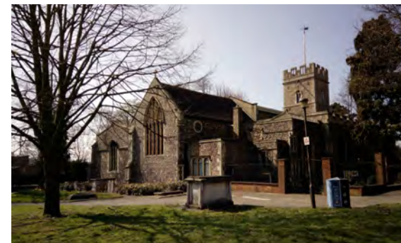
St Matthew's Church, eastern view, taken from Civic Drive.
