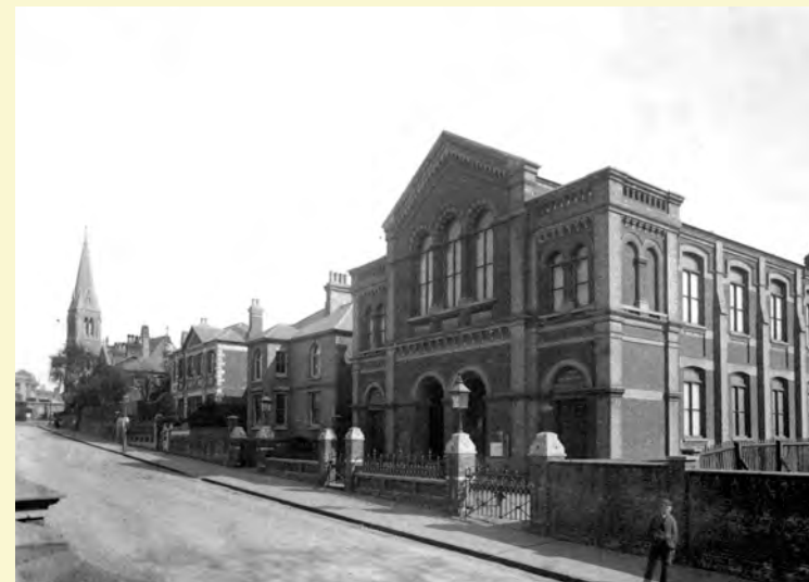
Burlington Baptist Church, London Road, looking north towards the Ipswich International Church at Barrack Corner, around 1880. The ornamental boundary walls which ran the length of London Road have since been demolished. (Image courtesy David Kindred).
