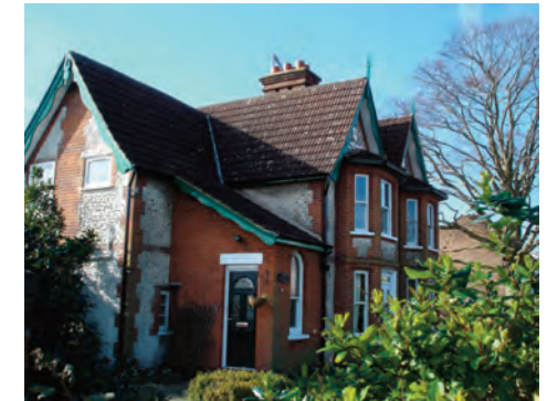
The earliest houses on the Cauldwell Estate, such as these examples on Freehold Road, have flint walling. Bricks were expensive in the mid 19th century, even though there were several brickworks in Ipswich.
