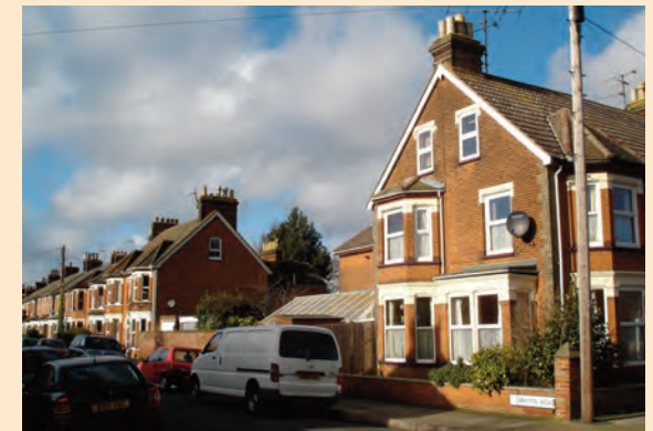
The well preserved scale and detail of street corners is an important aspect of the character area.
