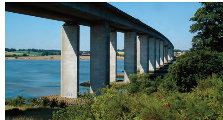
Orwell Bridge, completed 1982. At the time, the 190m main span was the longest pre-stressed structure in the world.
