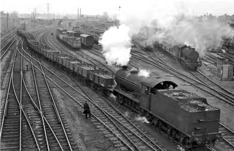
Railway lines and sidings, photographed from the London Road bridge looking towards Hadleigh Road. The railway arrived at Ipswich in 1846 with the first station at Croft Street in Stoke. The tunnel was built at the same time.
