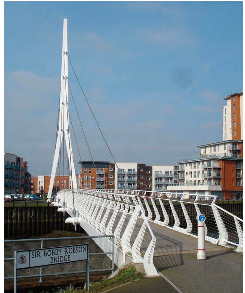
Above: Sir Bobby Robson footbridge. A 60m cable stay bridge, opened in 2009.
