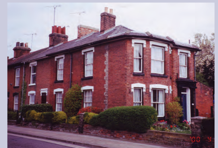
No 73 Christchurch Street
