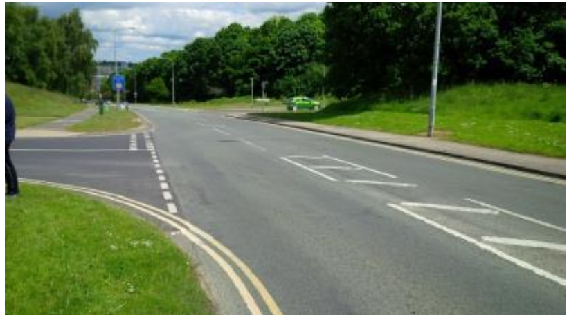
Birkfield Drive – potential for off-road provision
