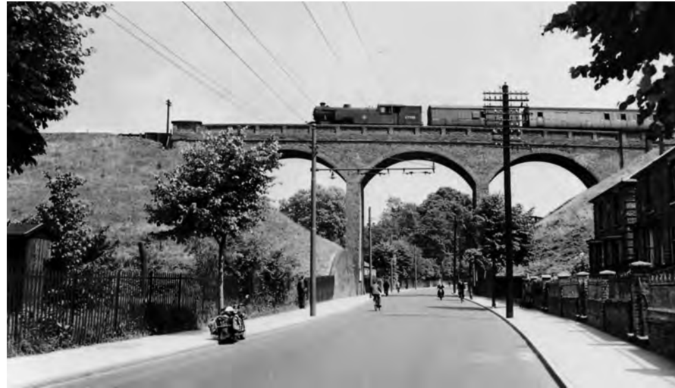
Spring Road viaduct. Part of the branch line built to Felixstowe and opened in 1877
