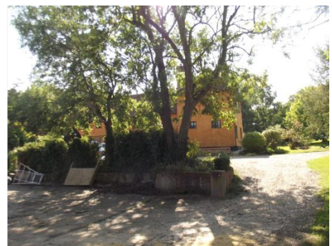
Fig. 21 Allen's House from bridle path
