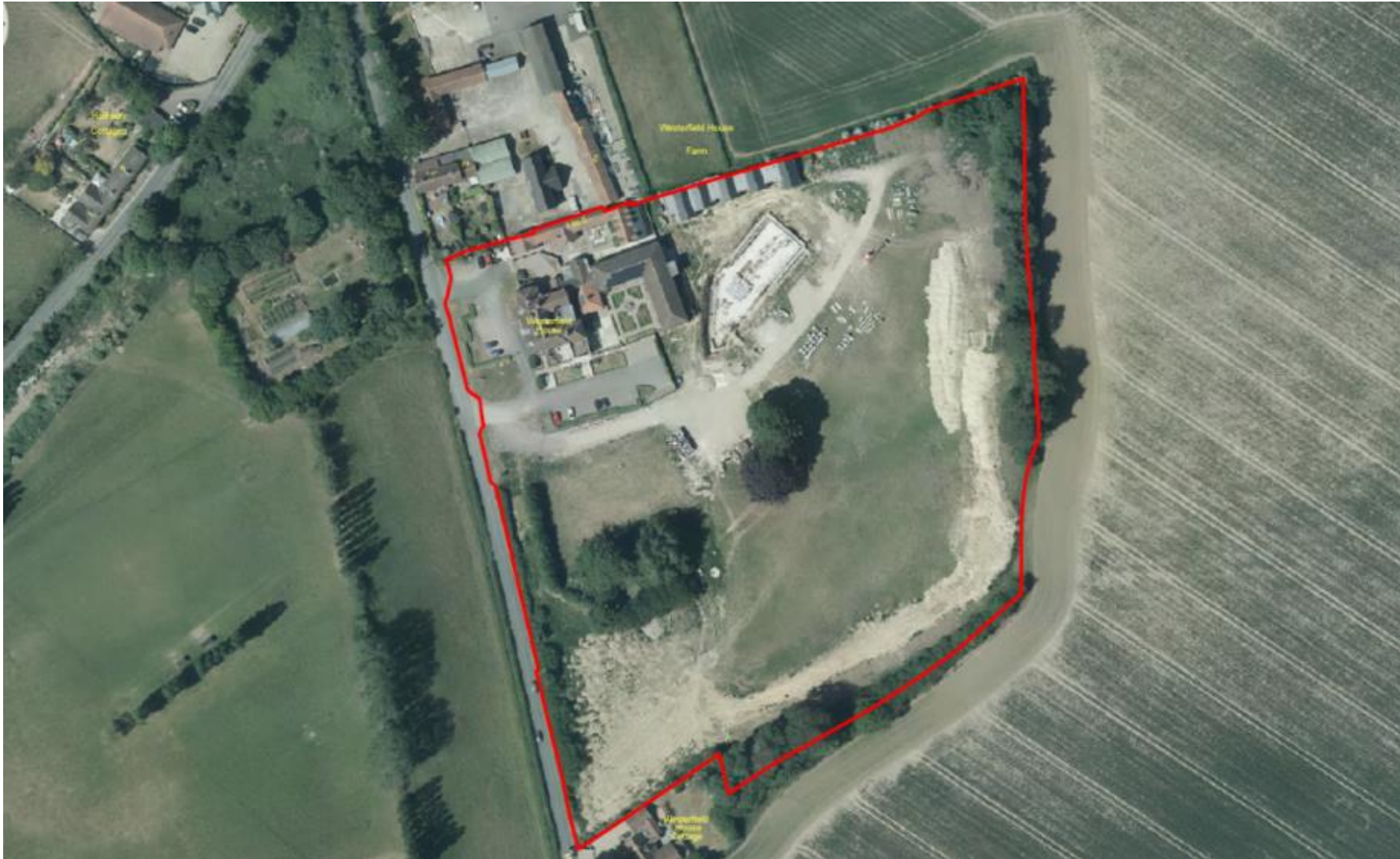
Appendix 18 – IP280 (Westerfield House) Aerial Photo Showing Commencement of Works (2020)
