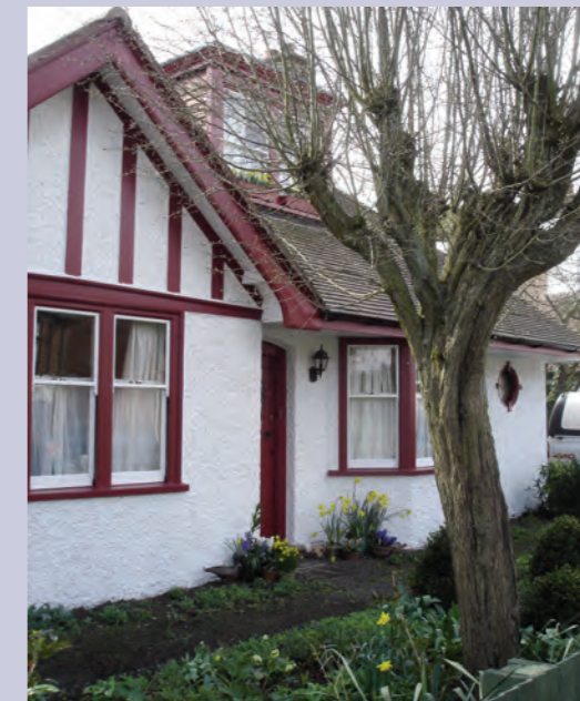
Bungalow – detail. Note the sash window design and the porthole window
