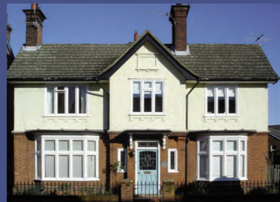
Top: Detached house on Tolworth Road
