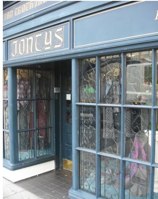
Fig 30 – Decorative iron grilles set behind the glass provide security, have a minimal impact on the appearance of the fascia and allow the display to be seen.
