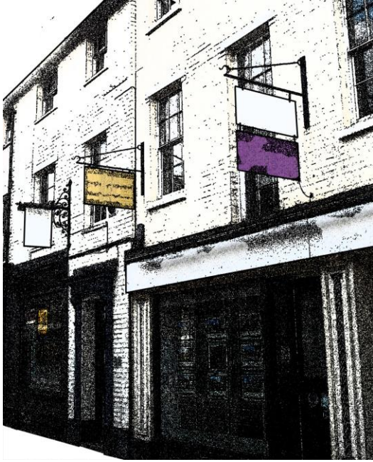
Fig 21 – These hanging signs are fixed too high on the façade, adding to visual clutter in the streetscape and blocking views of the original early 19 th century sash windows at first floor level.
