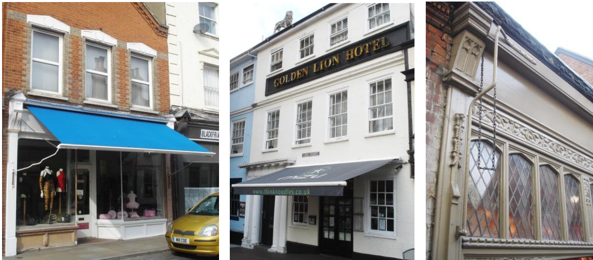
Figs 27-29 – A traditional retractable blind (left), a modern version (centre) and a blind retracted into its fascia box.
