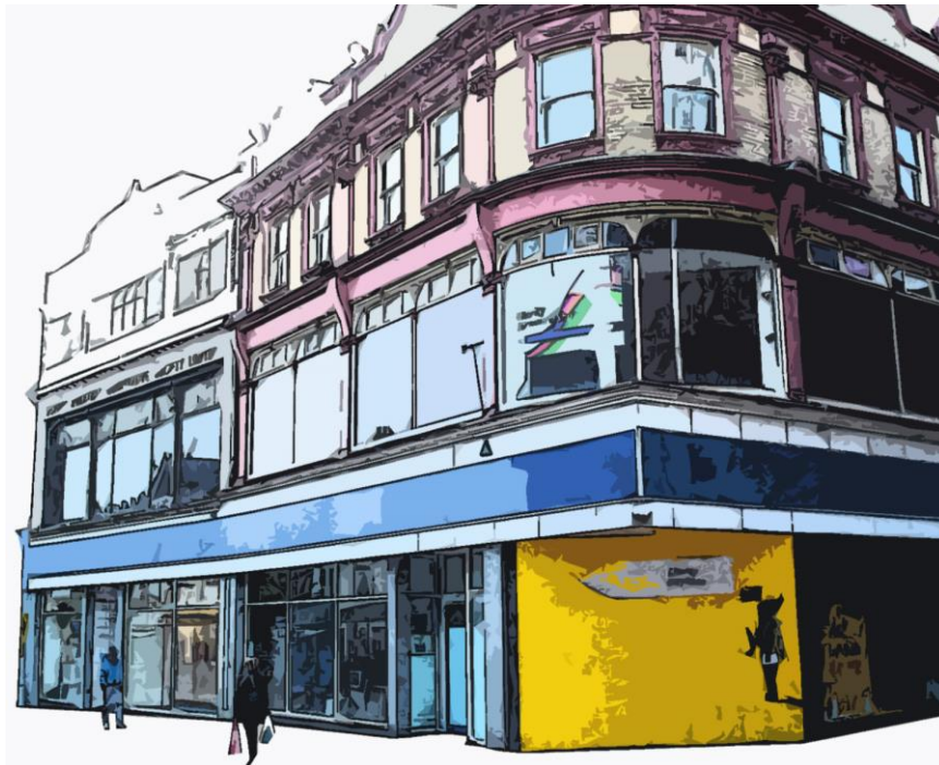
Fig 5 – The continuous fascia of this department store ignores the contrasting facades on the first and second floors above, which were built at different times and use different architectural styles and materials.
