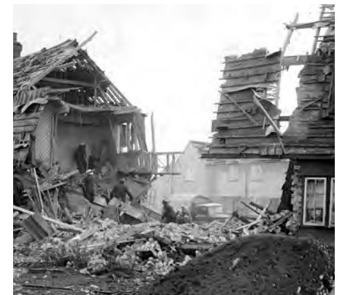
Bomb damaged houses at Romney Road following an air raid on 08.01.1941 – Photo courtesy of David Kindred
