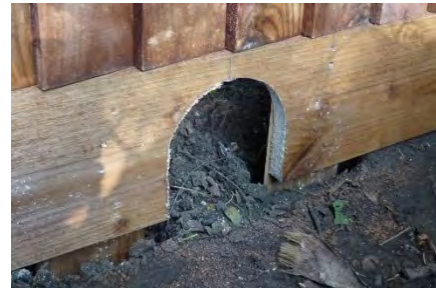
Fig. 7 - Example of permeable fencing.
