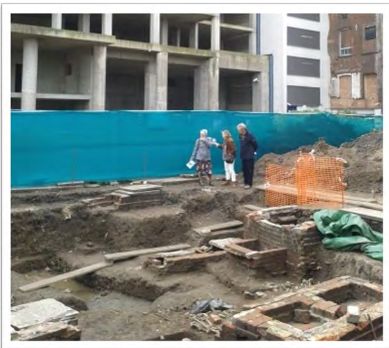
Figure 14: At St Mary at Quay church, several later vaults had cut through earlier layers. These were excavated and the pile design modified to place piles in these areas of previous disturbance where possible, to reduce some of the scope of archaeological excavations.
