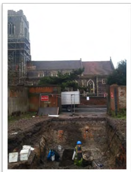
Figure 12: Evaluation at St Peter's Wharf. Urban trenches may be deep and may require stepping or shoring. Water may be an issue. (© Pre-Construct Archaeology).
