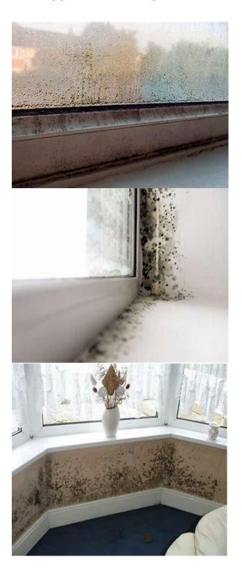
Condensation forms on cold surfaces, such as on reveals around windows. This is often the case in houses with solid walls.
