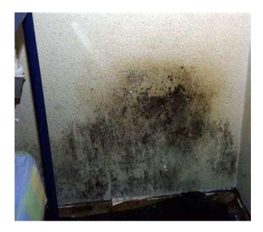
This is an example of an isolated patch of mould. This is very typically of where furniture is stored close to a wall and prevents air circulation.
