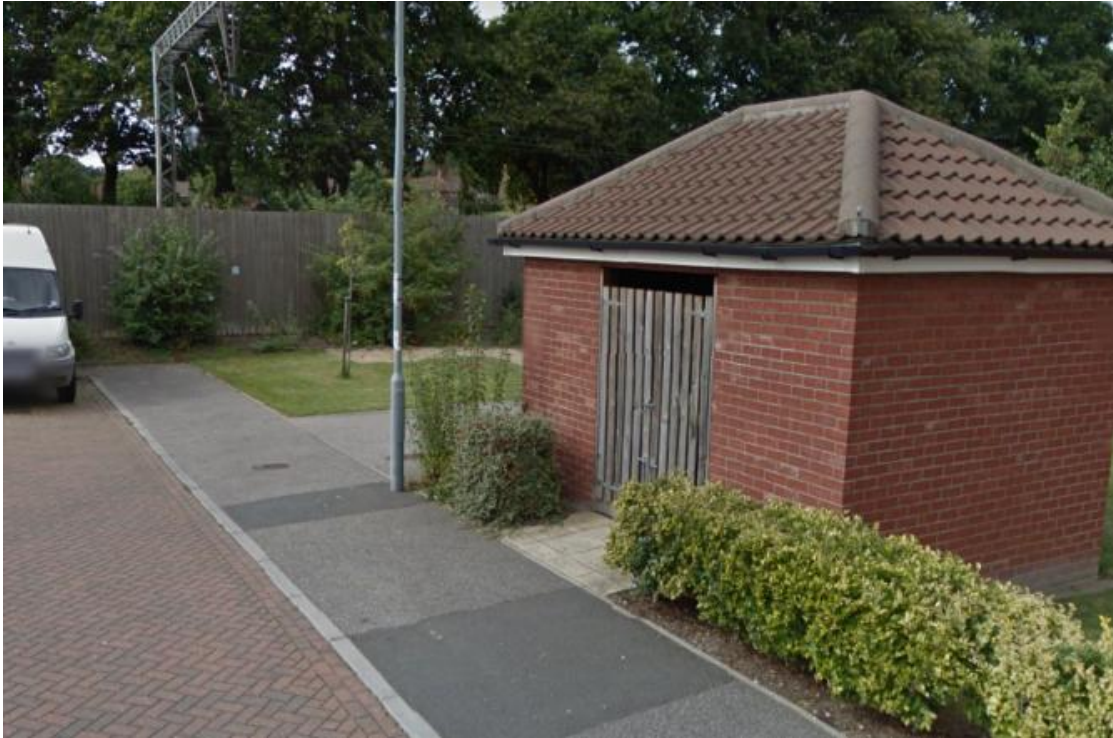
FIGURE 3 - GOOD ACCESS TO BIN STORE WITH DROP KERB
