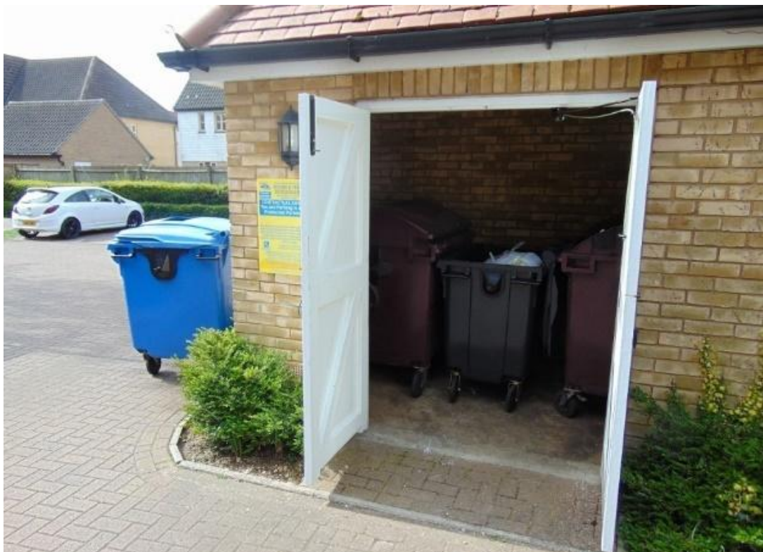
FIGURE 2 - POOR EXAMPLE OF COMMUNAL BIN STORAGE, CRAMPED AND DARK – NOT ALL BINS ACCESSIBLE, NOT LARGE ENOUGH TO INCLUDE ALL WASTE STREAMS
