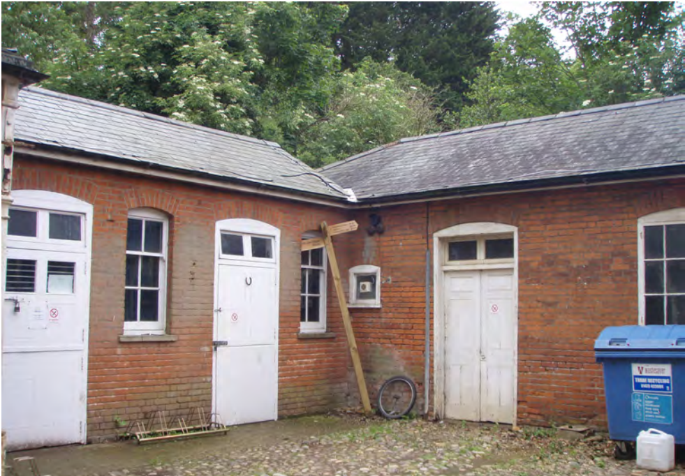
Photo 19 Southern elevation of Stable Block showing gaps beneath ridge tiles
