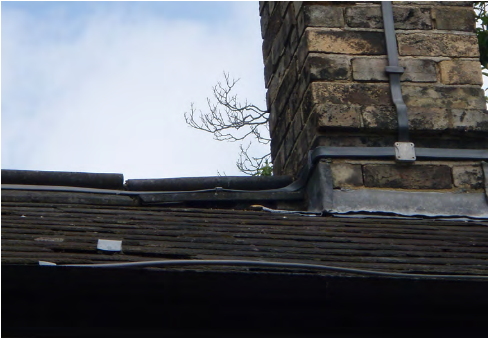
Photo 20 Gaps beneath ridge tiles and lead flashing on southern elevation of Stable Block
