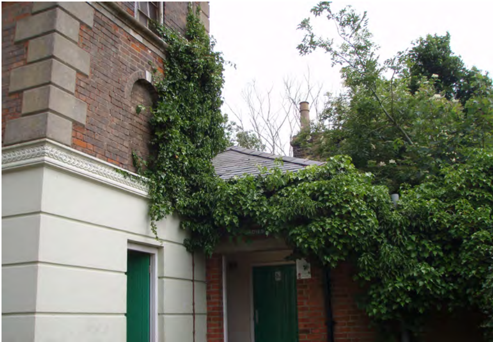
Photo 26 Toilet building with dense ivy on roof and western elevation
