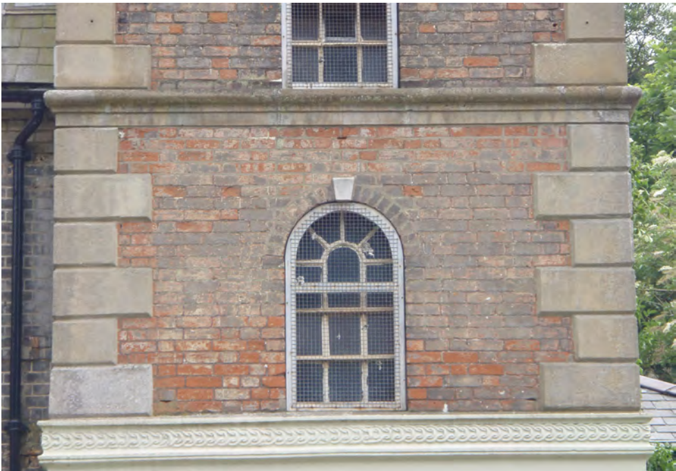
Photo 25 Northern side of clock tower showing gaps in mortar
