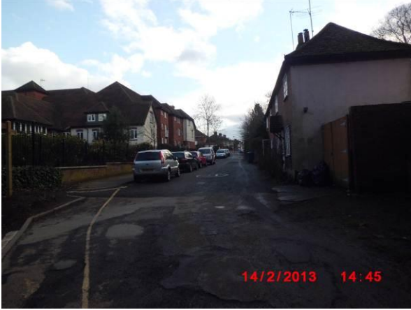
17. Current vehicle driveway and pedestrian footpath into Holywells Park from Cliff Lane entrance showing erosion and excessive parking.
