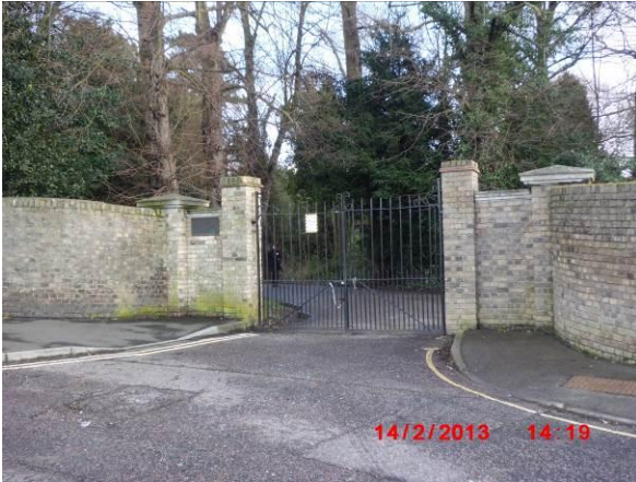
9. Entrance Gates at Myrtle Road.
