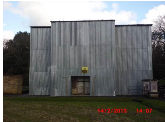
4. Western side of Orangery wrapped in corrugated steel for health and safety reasons.
