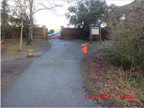
13. Nacton Road entrance showing brick piers, eroded pathway with encroaching vegetation.
