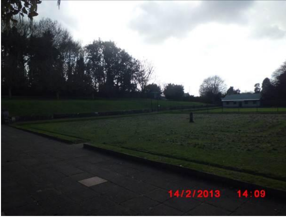
5. Current Maze at Holywells Park showing collapsing paving slab retaining wall.
