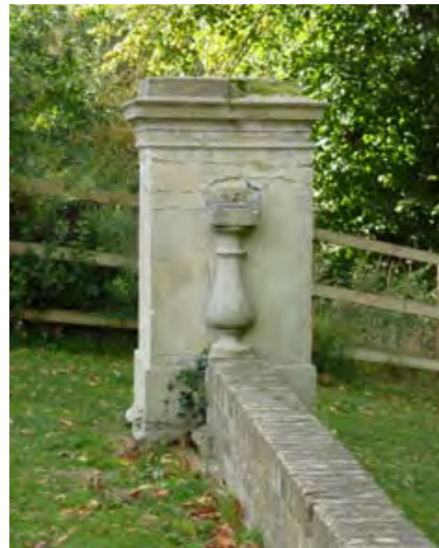
Missing balustrading.
