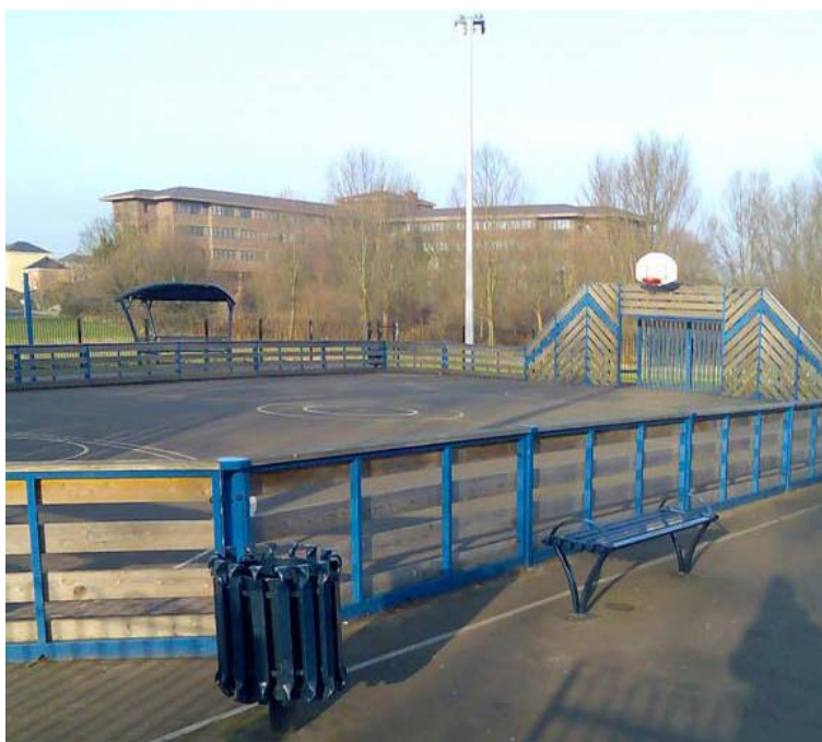
Figure 13.1 Alderman Road Recreation Ground MUGA
