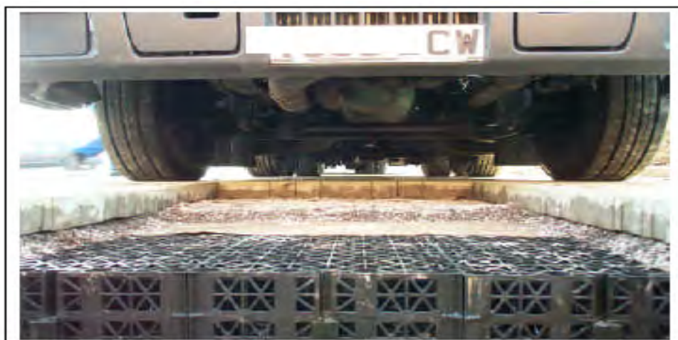
Plastic modular tank below a trial car park at Coventry University (CIRIA 2004)
