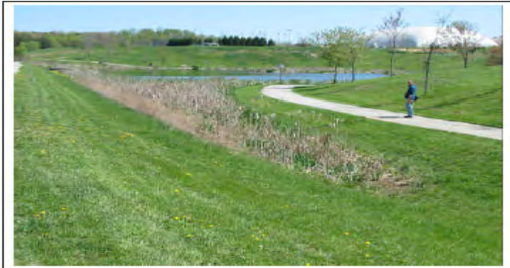
Swale integrated into landscape and retention pond (CIRIA 2004)
