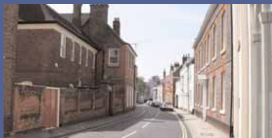
View down Lower Brook Street and Knapton House
