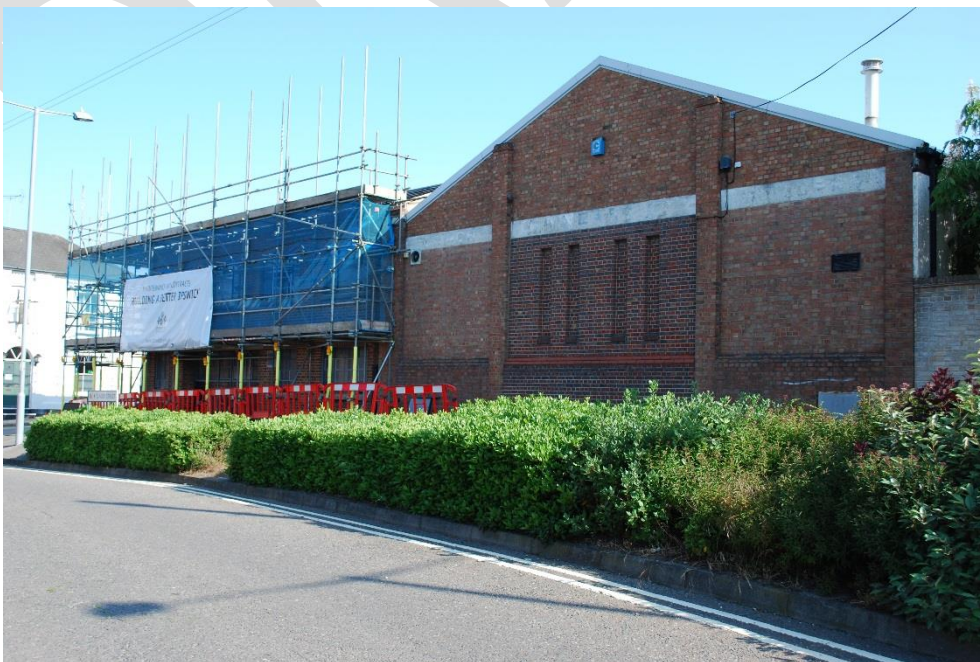
Figure 89. The former Nears coach works.
