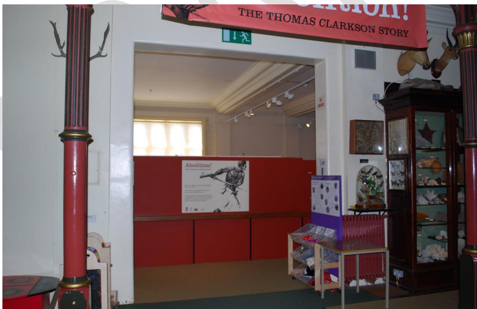
Figure 38. Opening to south range, formed 1924-6.
