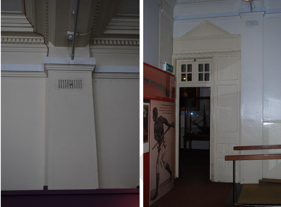
Figure 50. Redundant heating/ventilation flue Figure 51. Door to St George's Street wing, 1900.
