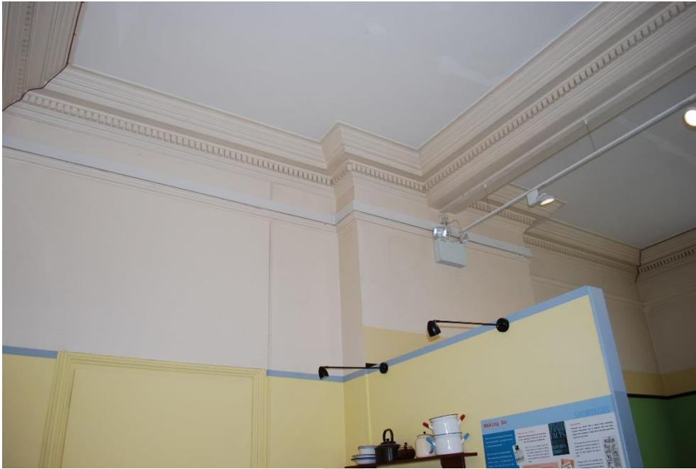
Figure 45. Former office for curator, showing blocked door and chimney breast.
