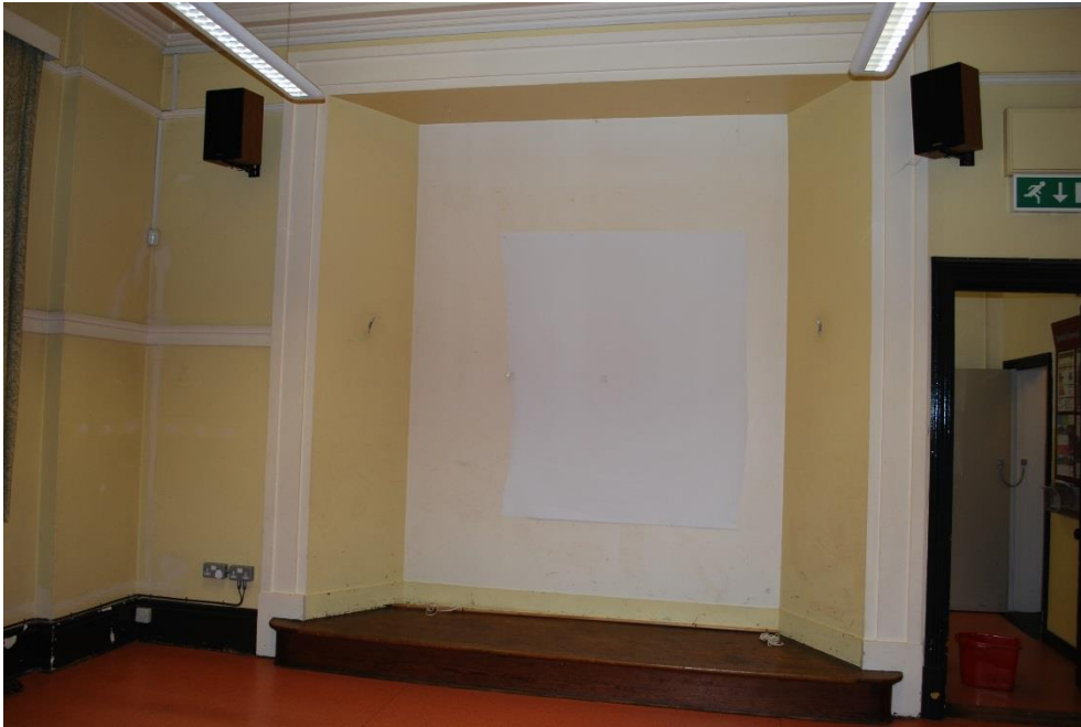
Figure 59. Art classroom, looking E with inserted wall and stage, 1930s.
