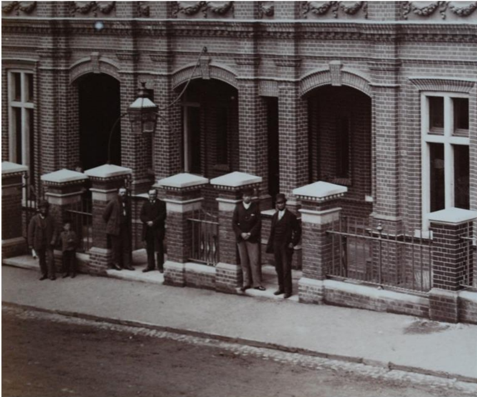
Figure 30. Detail of above, showing three historic entrances with gates and central lamp with overthrow.
