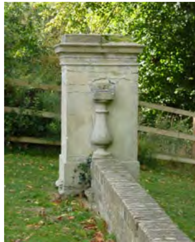
Missing balustrading.
