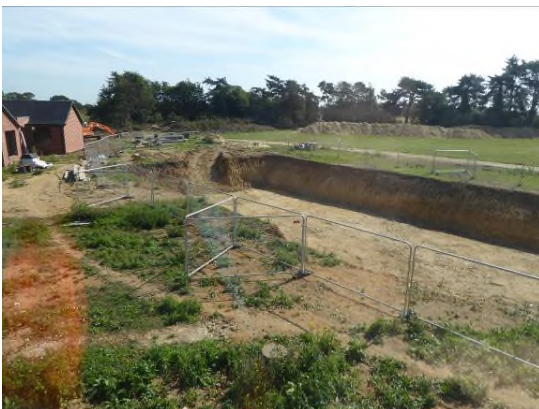
View east across recent excavations and new construction towards line of pines on boundary
