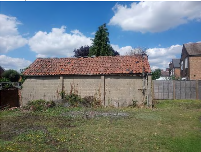
Outbuilding with potential bat roosting features
