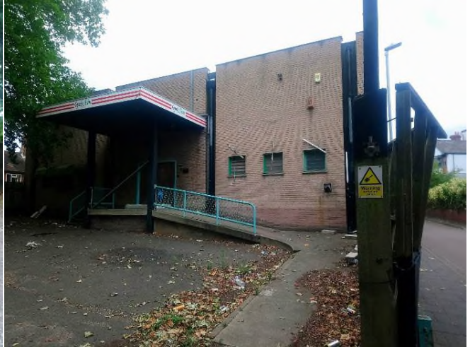
IP011a Disused gym
