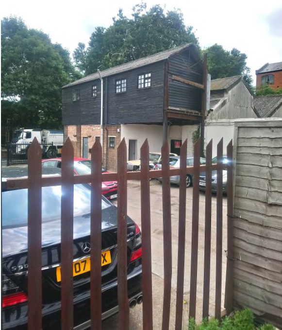
Building to south west
