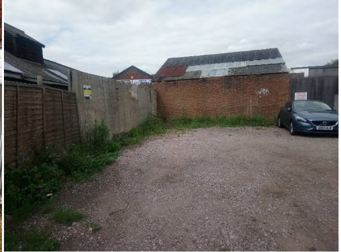
Gravel car park in south with sparse perimeter vegetation
