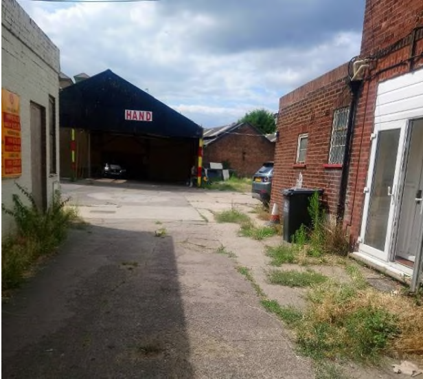
Hard standing with cracks in paving
