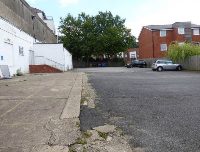
Car park behind Hope Church
