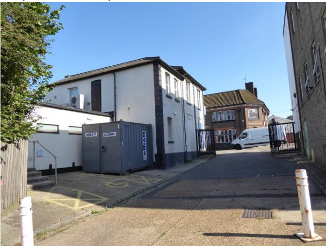
Building adjacent to Hope Church with bat potential and swift nesting potential
