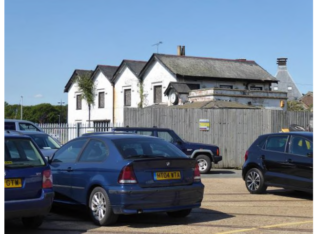
Building with bat and swift potential
