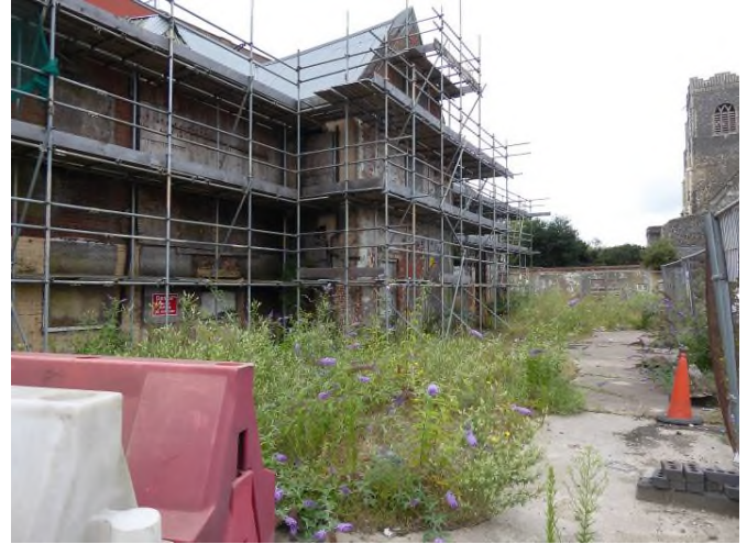
Disused building on southern part of site (Target Note 1)
