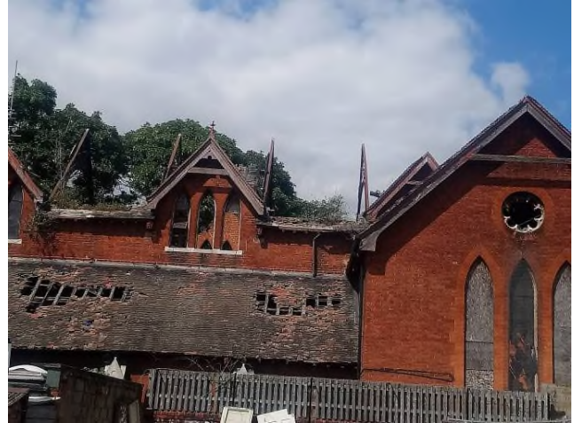
Burnt out church building to the north of the site
