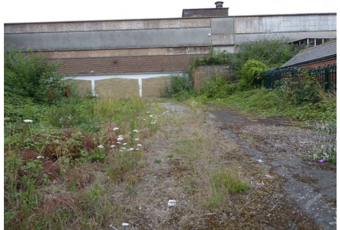
Low growing vegetation and disused building to the rear of the site
