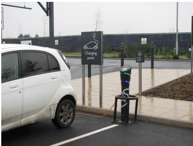
Electric charging point being used in the John Lewis Waitrose car park
