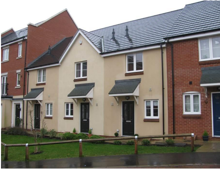
New homes at Meridian Drive, North-East Ipswich
