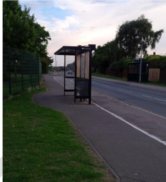
Bus stop bypass, with the cycle lane passing behind the bus stop. Note that whilst this is a good example of provision for cycling, ground based cycle symbols close to the bus stop area would help to make pedestrians aware of the cycle lane.
