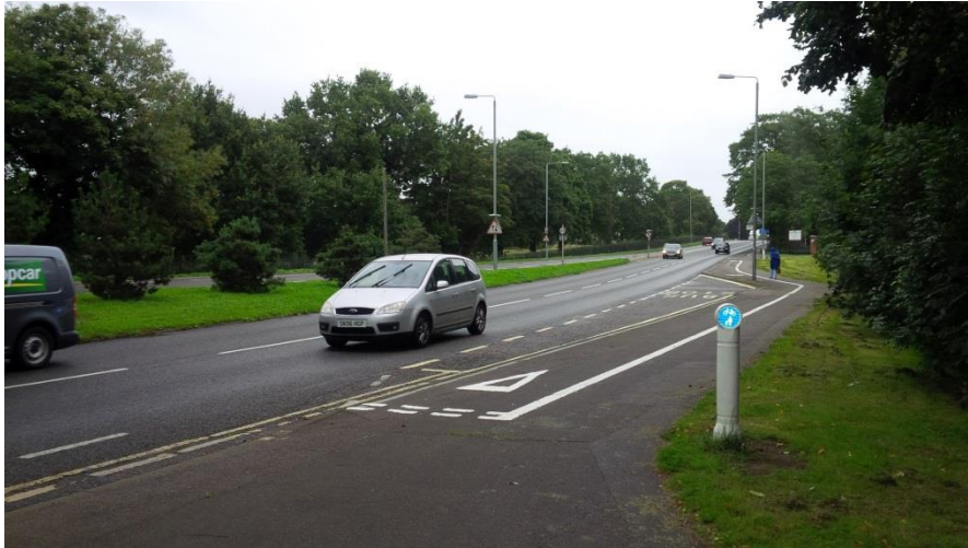
London Road – good example of off-road provisional although this is intermittent along the length of the road.
