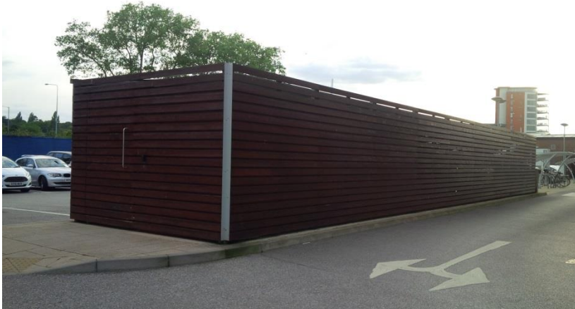
Example of secure cycle storage for large employers. This example is at Ipswich Borough Council’s offices at Grafton House.
