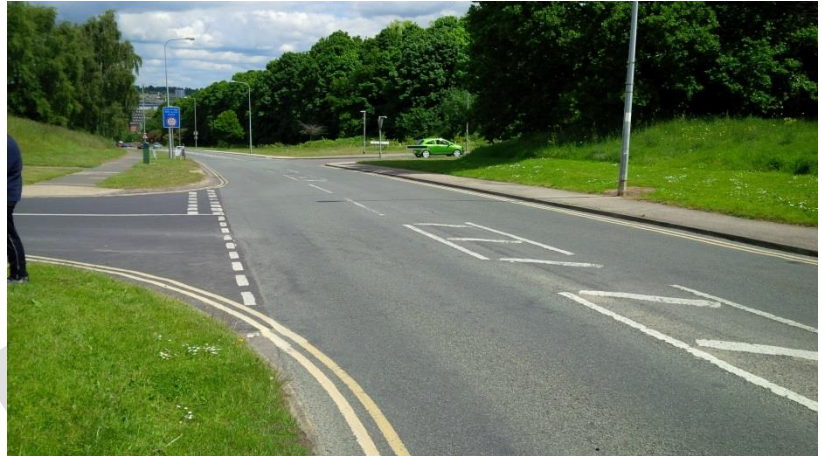
Birkfield Drive – potential for off-road provision
