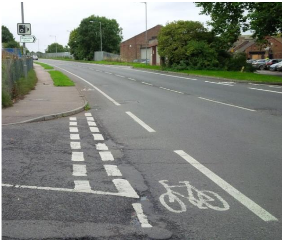
Above: On-road cycle lane providing no physical separation between the cyclists and vehicles. Where possible, physical separation from vehicles should be provided.
