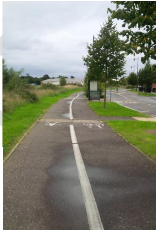
Right: This shows a good example of an off-road cycle path following the route of the road with a grass verge separates cyclists from vehicles.
