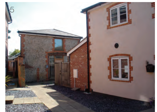
5 North Hill Gardens. A sensitive conversion of existing buildings which retains original fabric alongside appropriately scaled and detailed new build.
