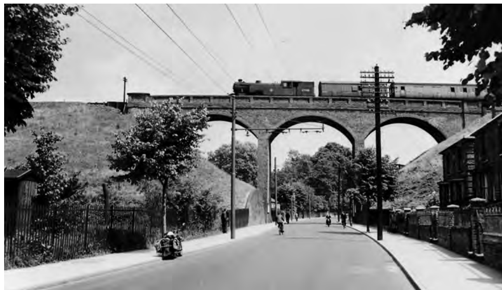
Spring Road viaduct. Part of the branch line built to Felixstowe and opened in 1877
