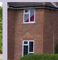
Dominant red brick character with brick work detailing.
