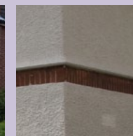
Red brick detail line through white painted render.
