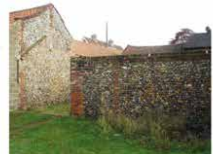
c. Red brick and flint outbuildings and walls
