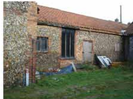
d. Farm outbuildings forming courtyard group. Red brick and flint. Clay pantile roof covering.
