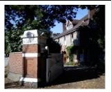
3 storey detached house with a principally roughcast rendered exterior, built in the 1920s. Red brick dressings frame the entrance porch and ground floor canted bay window, which include decorative terracotta plaques within the masonry. Timber sliding sash windows. Hipped clay tile roof with modest central dormer and larger side gabled dormer. Prominent red brick chimney stacks to either end of the building, penetrating the eaves level.
