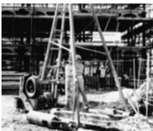
The drilling rig at the BRE environment building, used to drive a 70m deep borehole into a chalk aquifer
