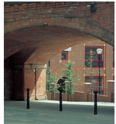
A new link has been punched through the railway viaduct - helping to stitch together the city centre and riverfront
