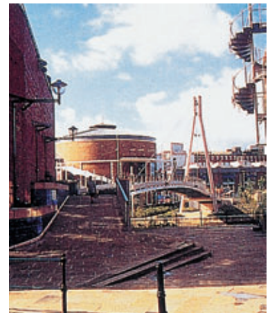
After: A new footbridge provides a direct route to the city centre
