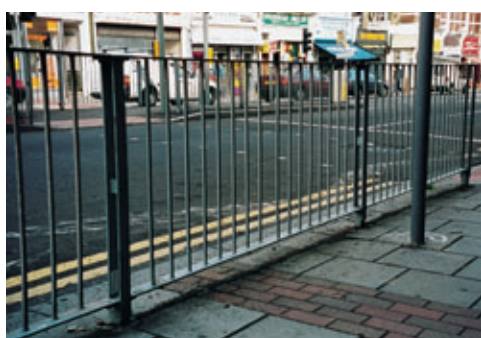
Sometimes facilities introduced in the name of 'pedestrian improvements' actually impede movement on foot and reinforce vehicular priority
