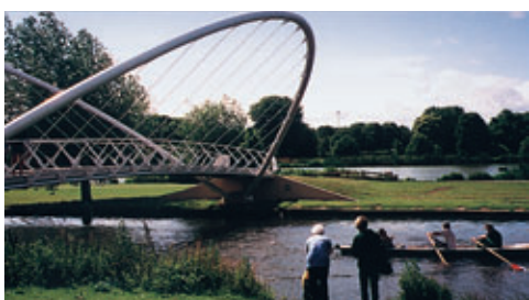
Ouse Bridge, Bedford (Architect: Chris Wilkinson)
