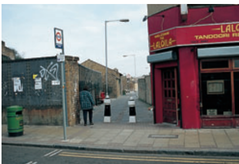
We should focus our efforts on improving routes to bus stops, yet all too often these are unattractive and intimidating.
