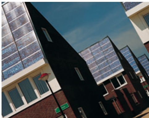
Urban design in the Nieuwland neighbourhood of Amersfoort, Holland, is centred on optimising solar potential
