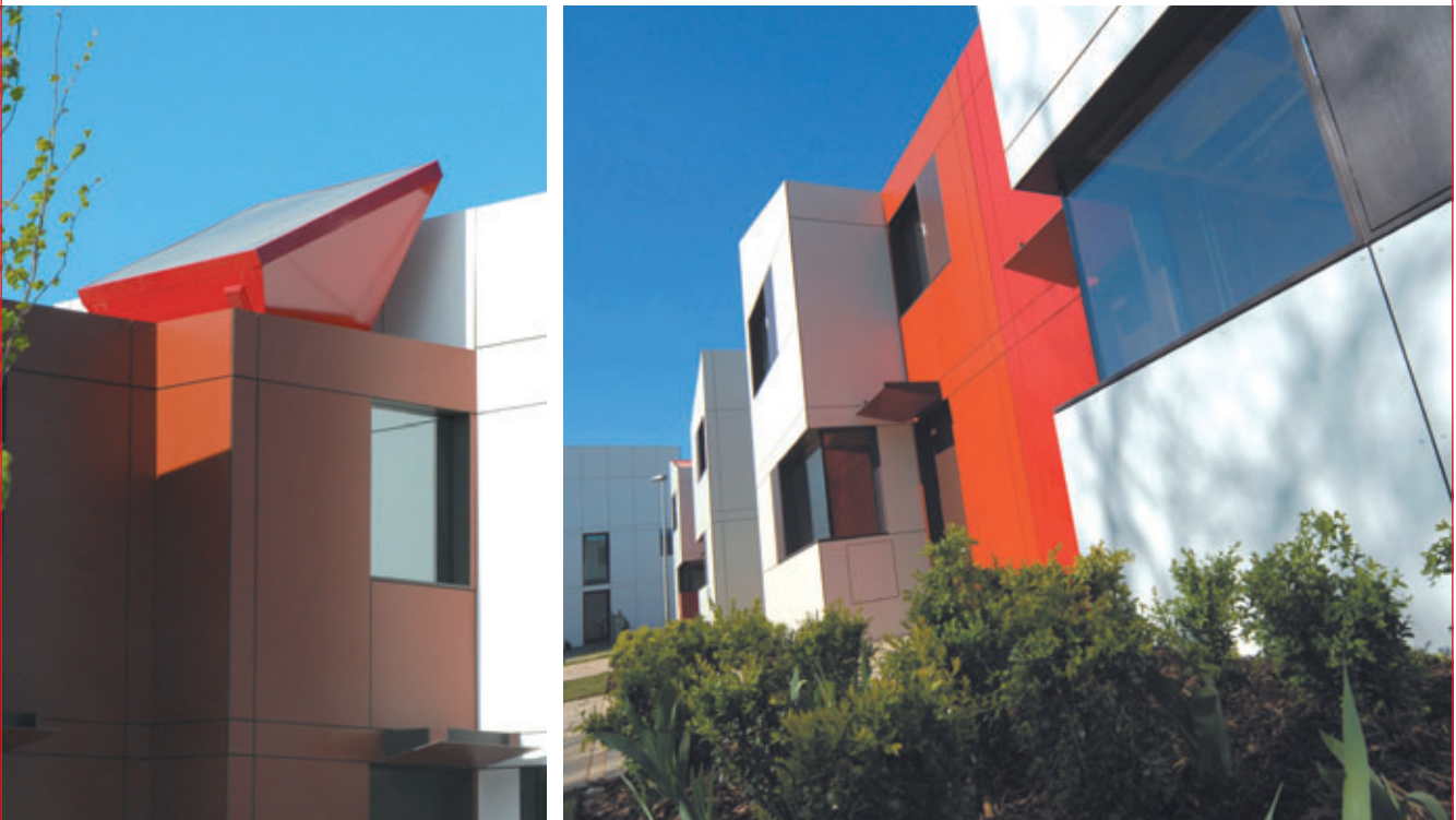
Designs for homes at Oxley Woods, Milton Keynes have shown how rigorous environmental standards can help to generate exciting designs through off-site prefabrication, reduced on-site construction costs and features such as an 'Ecohat' for ventilation, photovoltaics and solar thermal heating.
