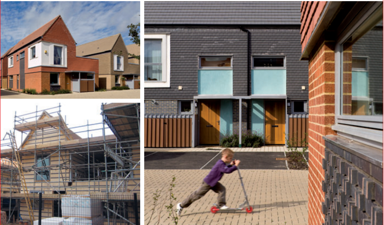
Homes using the polarwall insulated concrete formwork system have been constructed alongside those using traditional block construction, which enables accurate comparison of the construction process and lifetime performance.
