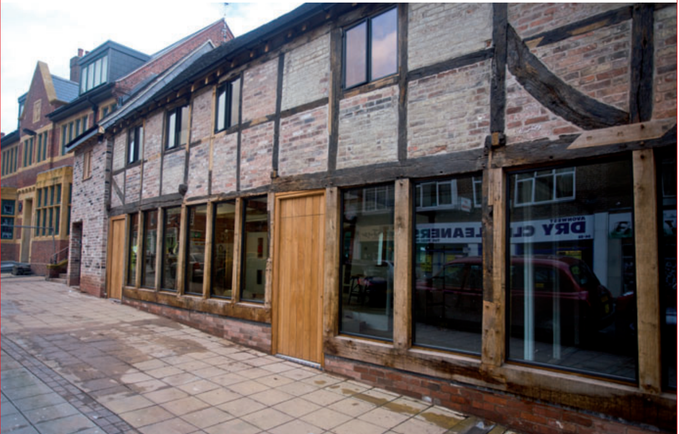
The Far Gosford Street regeneration project brings new life to historic buildings. Over forty buildings have benefited from investment to date, ranging from minor frontage improvements, façade restoration to full refurbishment, such as this 17th century timber-framed building at number 121-124.
