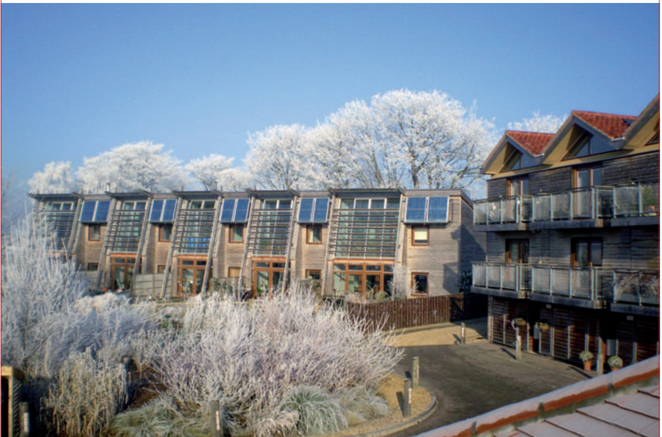
The northern and eastern terraces have distinctly different designs that reflect the position of the buildings in relation to the sun and view across the river.
