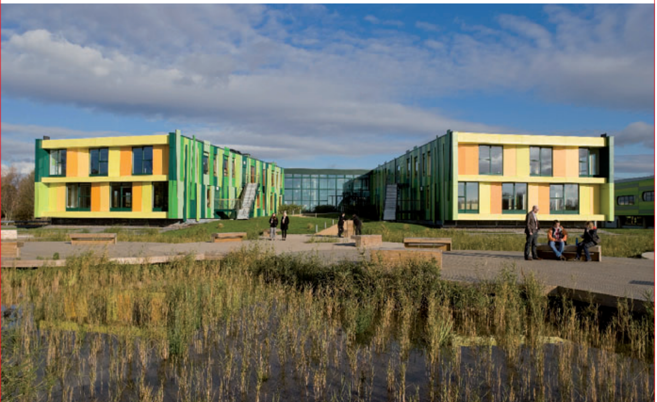
Blueprint's extension to Nottingham Science Park is designed to visually and physically link the site to the surrounding landscape.
